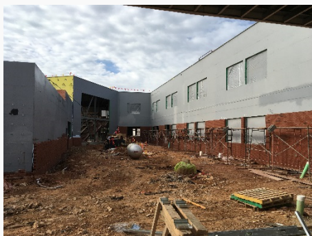
Brick Install at Courtyard
