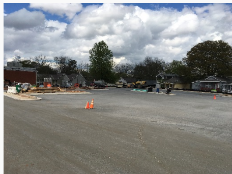
Preparing Parking Lot and Drive for Binder and Asphalt
