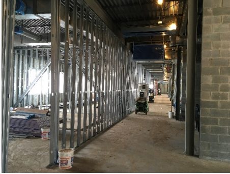
Interior Framing at Upper Level
