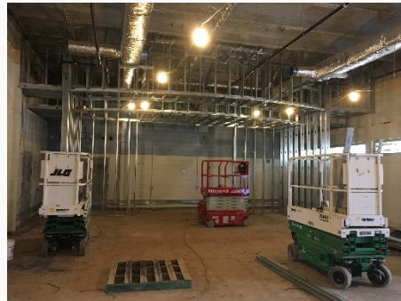
Interior Framing for Stage at Auditorium
