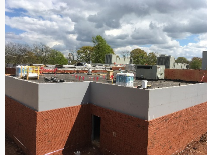
Completing Air Barrier & Brick
