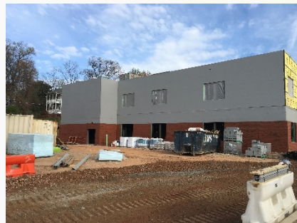
Exterior Framing, Sheathing, Air Barrier, & Brick
