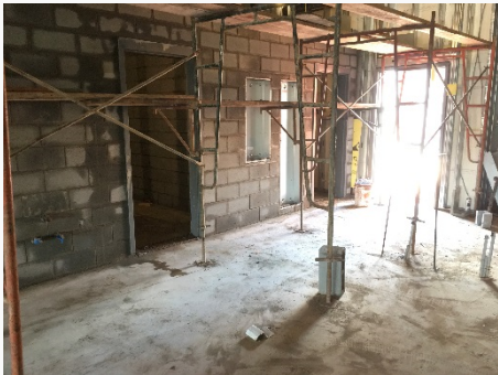
CMU Walls, Door Frames, & Elec. Panels at Kitchen
