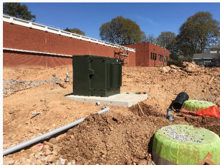
Main Electrical Transformer
